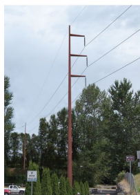
Sample Pole and Wiring Configuration Pole heights will range from 95 ft to 125 ft : energizeeastside.com/design
