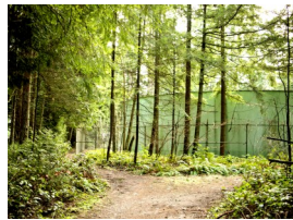
Pike's Peak Water Reservoir
